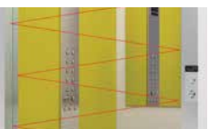
Photoelectric curtain for safety and comfort of passengers
